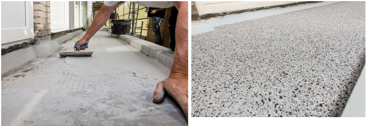
Figure 10: Installation of the EZA system on balconies (left), finished surface (right), Rotterdam 2014
