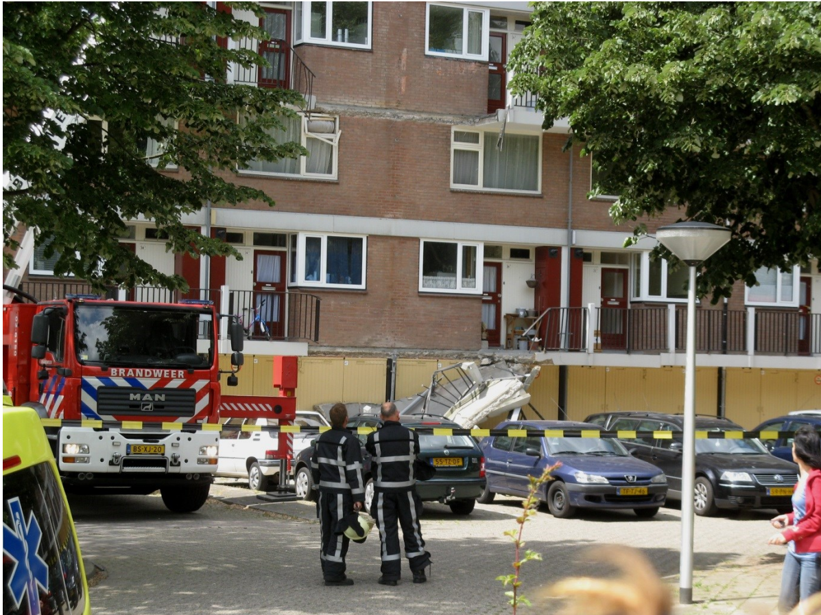
Figure 9: Failing cantilever slabs (The Netherlands, 2011)
