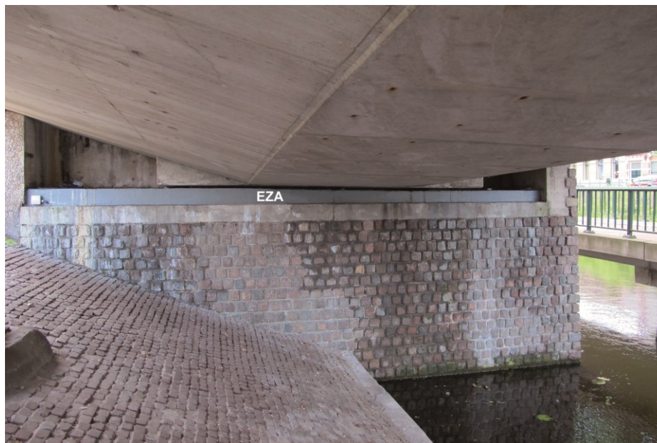
Figure 8. EZA installed on the beams supporting the bearings of the Hubertus viaduct in The Hague
