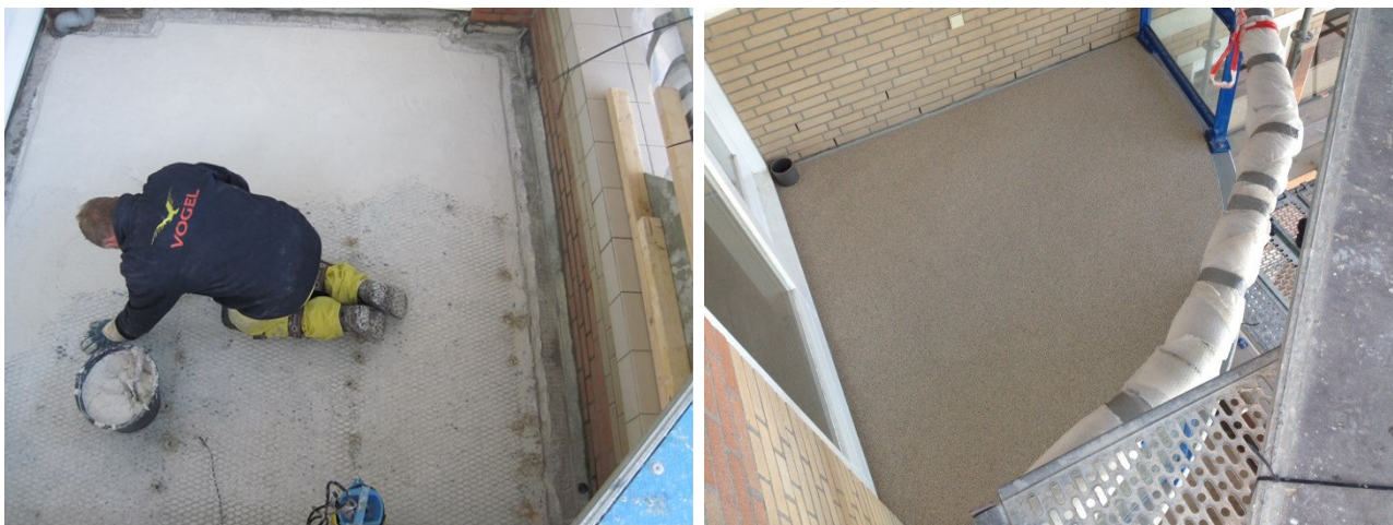
Figure 11: Installation of the EZA system on balconies (left), finished surface (right), Egmond aan zee: 2014
