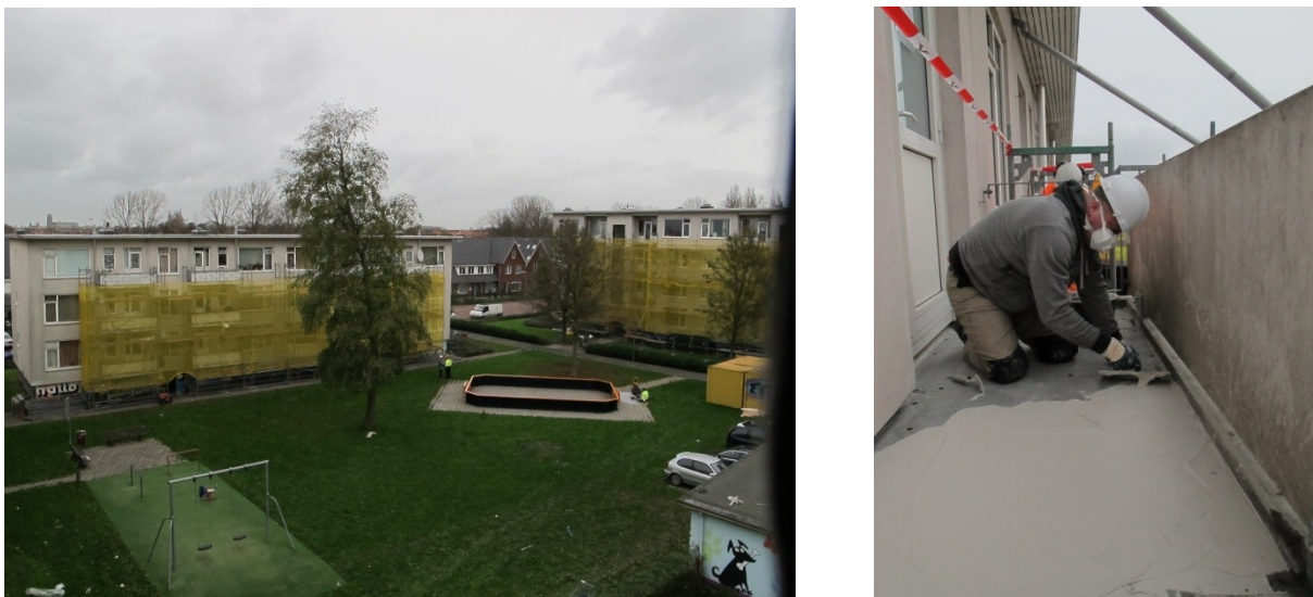
Figure 12: Installation of the EZA system on a total of 400 balconies of apartment buildings (left), finished balcony surface (right), Dordrecht 2015
