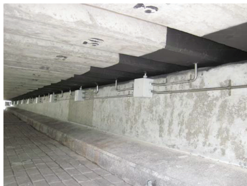
Figure 1. As-built CP system with conductive coating and decentralized power supply and monitoring units.
