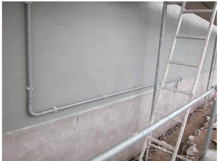
*Figure 12: Installation of the titanium ribbon mesh anode on the sustaining wall above and below the ground line, embedded into shotcrete, left picture zone 1. B2134; right picture zone 4, B2136.*
