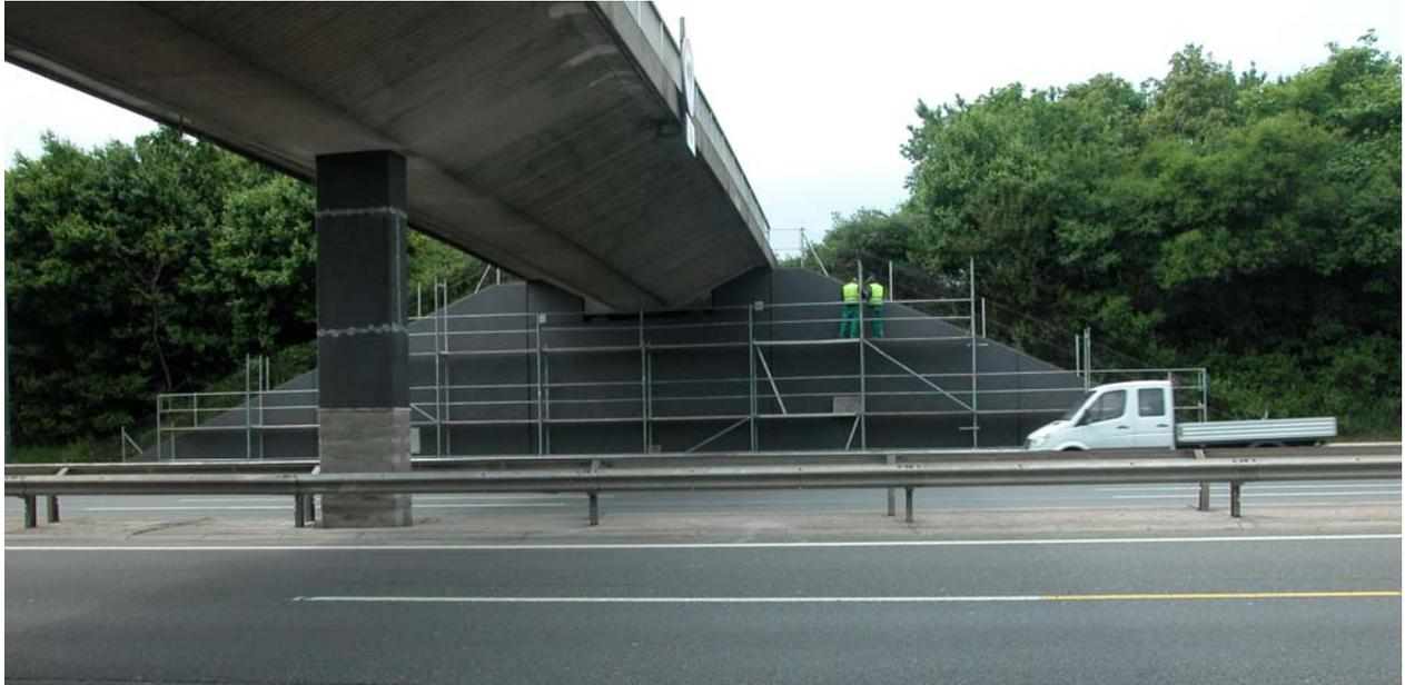
*Figure 8: Installation of the CAS-Composite Anode B2134: bridge column – zone 3, CAS-CNP primary anode on 1<sup>st</sup> layer of CAS-T<sup>+</sup> coating; abutment – zone 2, second layer of CAS-T<sup>+</sup> coating embedding the CAS-CNP primary anode.*
