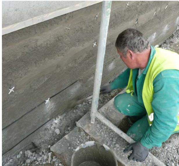
*Figure 11 Titanium ribbon mesh anode on the sustaining wall above and below the ground line, B2134, zone 1.*
