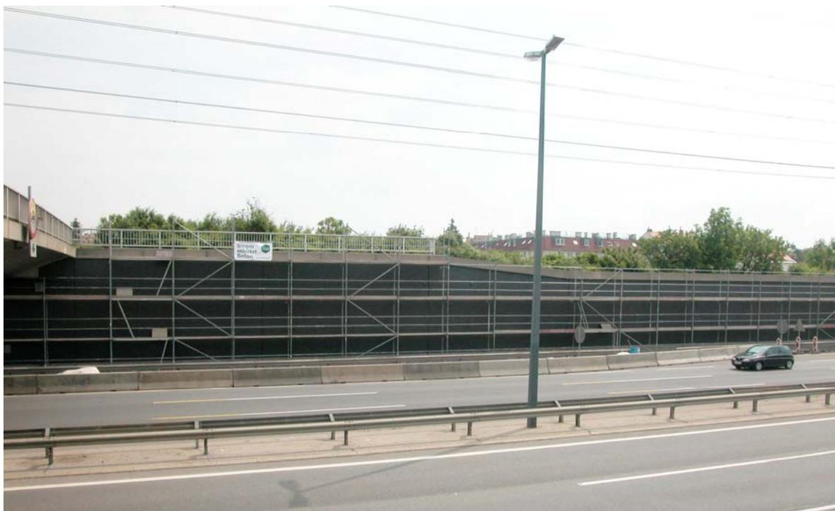
*Figure 7: Installation of the CAS-Composite Anode in Zone 1 (sustaining wall, B2134 RF Stockerau) – 1<sup>st</sup> layer of CAS-T<sup>+</sup> coating.*
