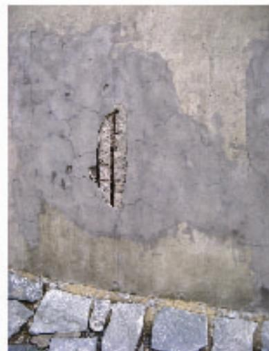
*Figure 3: Visible damages to the sustaining wall of the bridge B2134.*
