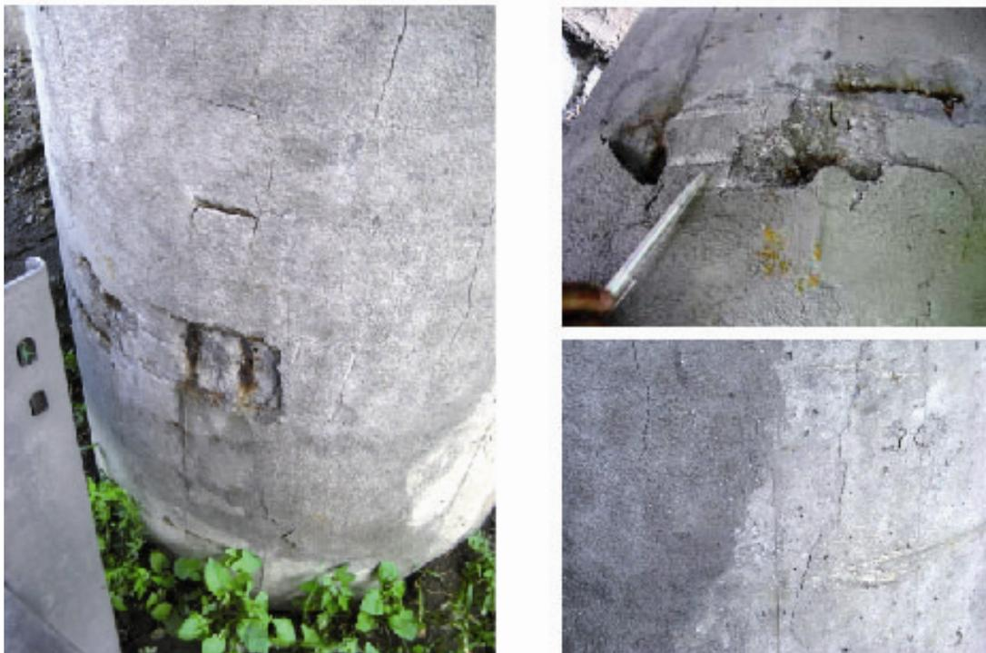
*Figure 4: Visible damages to the bridge columns of the bridge B2136.*
