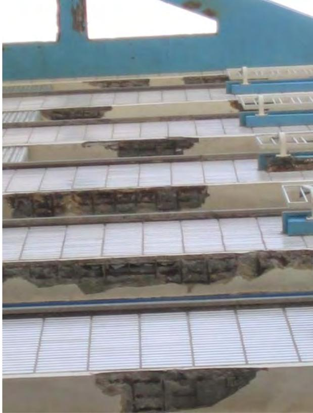
Figure 1: Spalling and disbondment of the concrete cover due to steel rebar corrosion.
