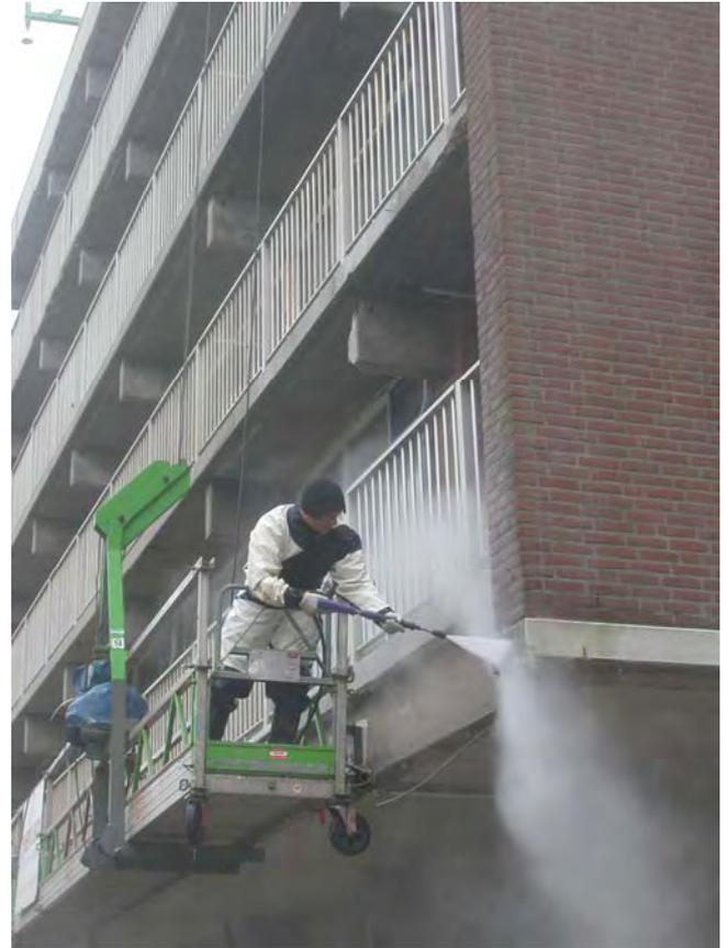
Figure 10: Concrete surface preparation and cleaning by high pressure water jetting.
