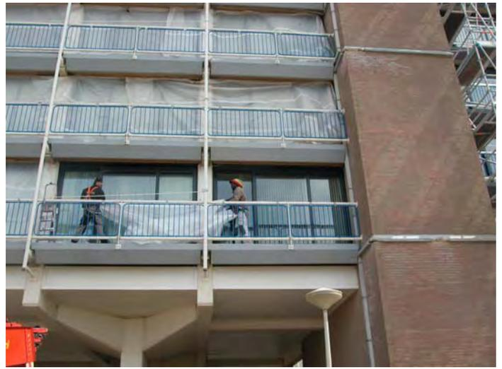
Figure 6: Covering the windows with plastic sheets before repair and installation works start.
