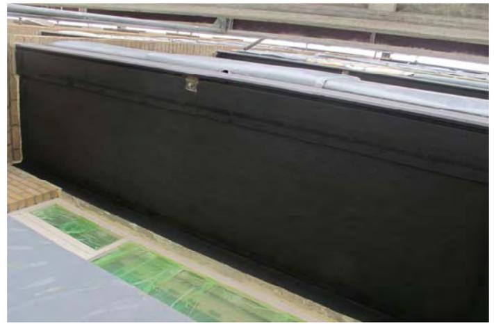
Figure 14: Underside of balcony coated with the CAST<sup>3+</sup> composite anode paint.
